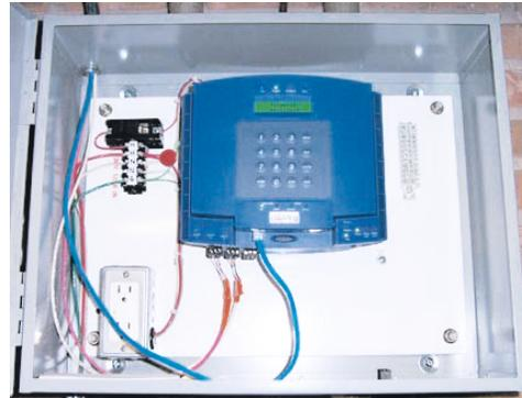
*The eBuilding Network Controller, one of nine installed at District 63*
